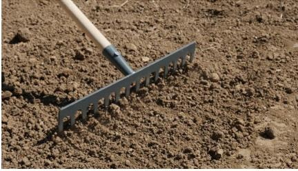
Rake the soil to begin to level it out, remove any rocks or debris that you find. To avoid problems with excess run-off, make sure that any site grading you do allows water to flow *away* from the house. Now, use a lawn roller filled 1/3<sup>rd</sup> full of water over the area to firm and settle the surface, and reveal any areas which may require more soil.
